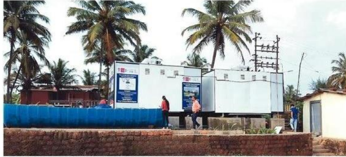
The facility makes it possible to reuse sewage for gardening, car-washing and toilet flushing purposes
